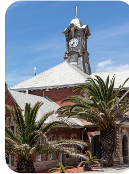
Muizenberg's historic station
